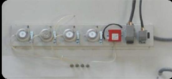
USING A SET OF PRESSURE READERS THAT SEND SIGNALS TO THE PLC WE ARE ABLE TO KNOW DIFFERENT MAINTENANCE NEEDS OF THE EQUIPMENT WITH HIGH ACCURACY AND ALSO TO GIVE POSSIBILITY OF SENDING A SIGNAL TO A FREQUENCY VARIATOR THAT ACTS DIRECTLY IN THE EXTRACTION MOTOR AND KEEPS **CONSTANT AIR FLOW KEEPING SPEED EXACTLY AT CORRECT MEASURE** WITHOUT DEPENDING ON THE CLEANLESS OF ANY OF THE THREE FILTERING AREAS.
